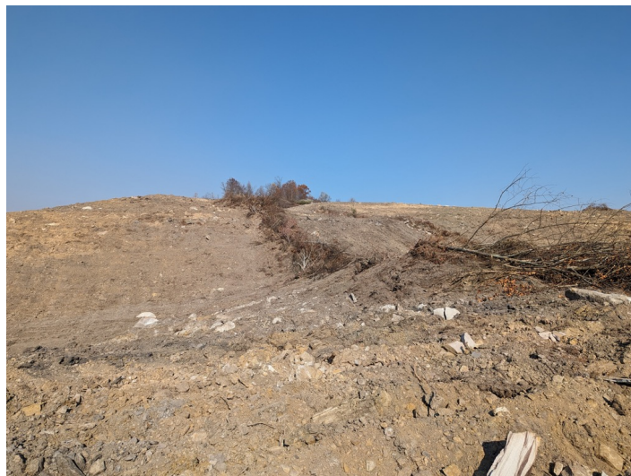
Figure 3. Unwanted vegetation and the top three inches of soil are pushed into berms within the project area and at the perimeters. They serve as habitat for insects, birds, amphibians, reptiles, and mammals as well as helping preventing offsite erosion and sedimentation of downstream watersheds.
