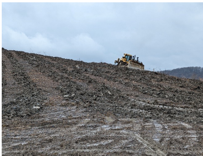
Figure 4. After the vegetation and the top three inches of soil is removed (left), a large bulldozer equipped with two, three foot ripping shanks decompacts the soil (right).
