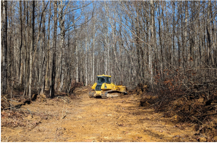
A small bulldozer fells unwanted trees on the haul road.
