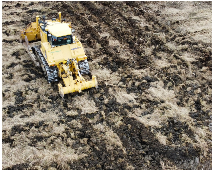
Site preparation is conducted using a Komatsu 155 with dual ripping shanks.
