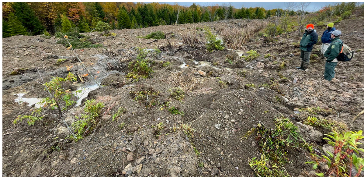
Top: Aerial view of the ponds before work begins on their removal. Above: Post removal landscape in an area where one of the ponds was decommissioned.
