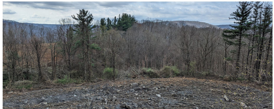
Before (top) and after (above) site prep at the Hylton Strip restoration area in the NRG.
