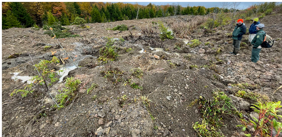
Top: Aerial view of the ponds before work begins on their removal. Above: Post removal landscape in an area where one of the ponds was decommissioned.
